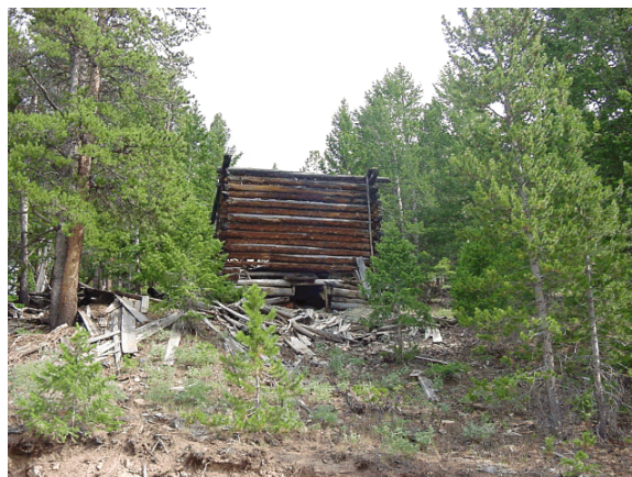
Figure 3. View of the old ore bin at the Blue Jay mine.
